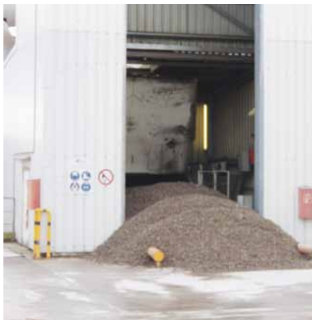
Unloading zone for RDF pellets.
